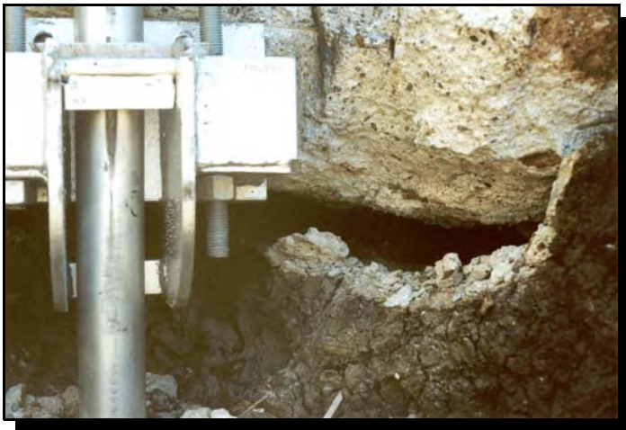
The lift is complete
