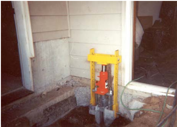
The pier is set and ready for the lift.
