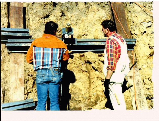
Testing and Pre-stressing Anchors
